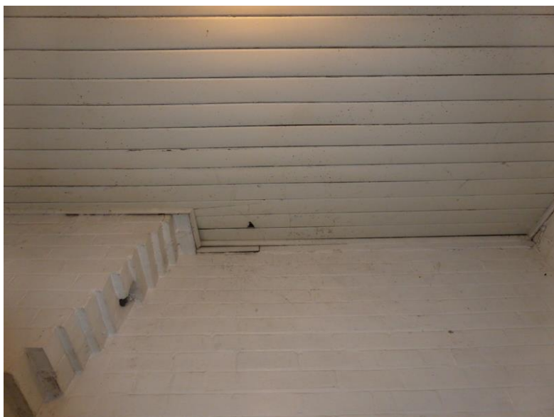
Figure 47: Timber ceiling of the Laundry. The back wall of the chimney of the Kitchen fireplace is evident.
