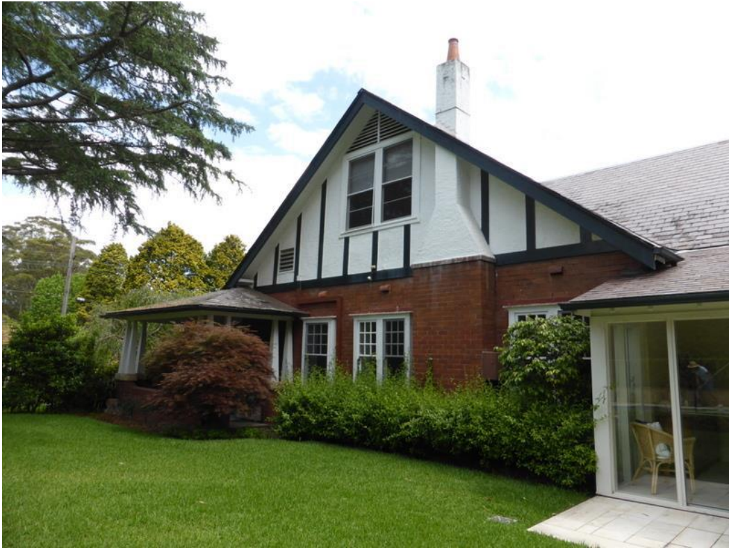
Image 4 – Photo eastern facade (Source: Kate Higgins Heritage Consultant)
