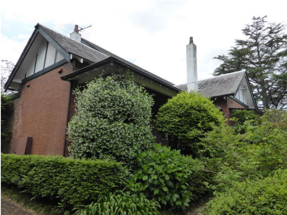
Image 5 – Photo western façade (Source: Kate Higgins Heritage Consultant)
