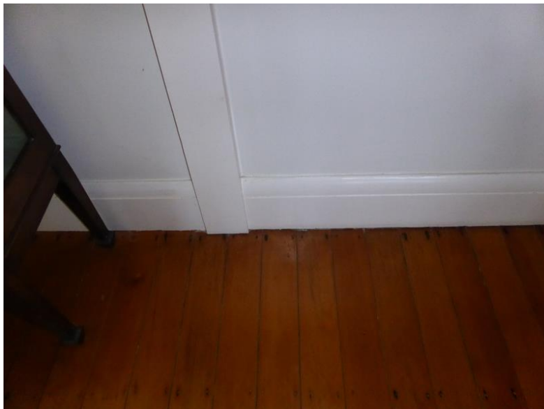
Figure 46: Simple timber skirting.
