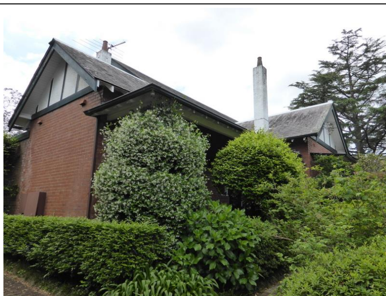
Figure 31: The western facade of the house showing the small gable which terminates the roof over the bedroom bay. The chimney of the existing living room is evident.
