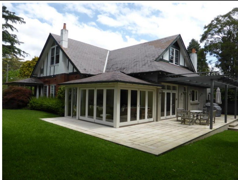
Figure 27: The rear and eastern side of the house. The rear gable roofed extension of the original hipped roof is evident. The windows in the gables are alterations to the original. The rear terrace and painted timber pergola are modern changes as are the glazed doors to the sunroom.
