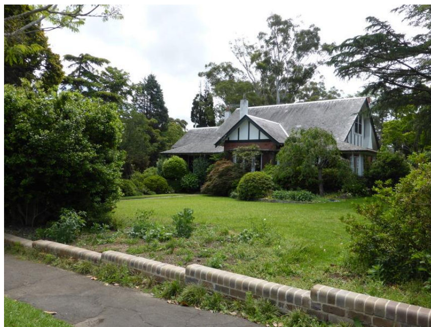
Figure 49: View of the front garden from the footpath showing the front lawn and garden bed immediately in front of the house. The front fence was original a timber fence.
