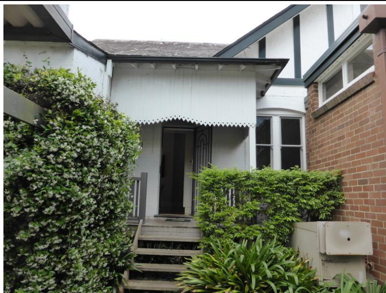
Figure 30: The back verandah and large western gable which terminates the main roof. The wall of the modern bathroom addition is evident on the right and the laundry on the left. The lightweight carport is just visible on the left.
