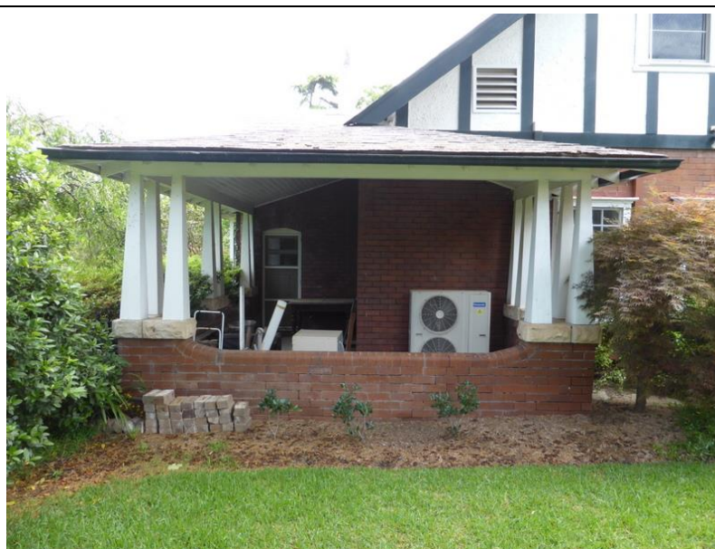
Figure 32: The verandah which wraps around the south-eastern side of the house. The tapered timber posts sitting on sandstone bases support the roof.
