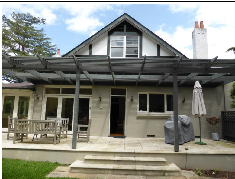
Figure 28: The rear (northern) facade of the house. Most of this façade has been altered from the original. The kitchen chimney is evident.
